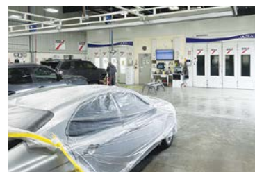
The well-equipped facility features drive-through Blowtherm paint booths and heated down-draft paint prep stations.
