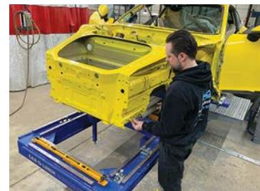
**Technician Mike Krason is shown reassembling the front end of a 2020 Porsche 911 Carrera S. The severe structural damage required replacement of the entire front end. CCC<sup>®</sup> refers to the part as the front inner structure.**
